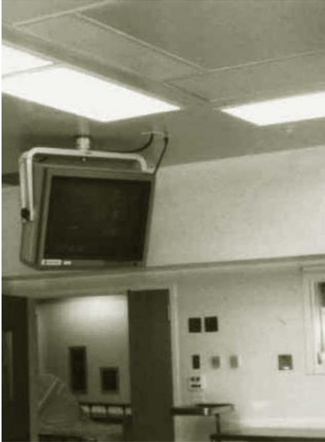
**Figure 5 depicts special fluorescent lighting whereby half of the lights can be turned on or off as needed. Note that excessive lighting causes glare on the remote monitor, making it difficult to see.**
