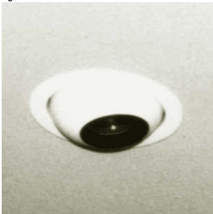
**Figure 4 depicts a special procedure light (spot light) that can be adjusted for use by the scrub nurse or anesthesia staff.**
