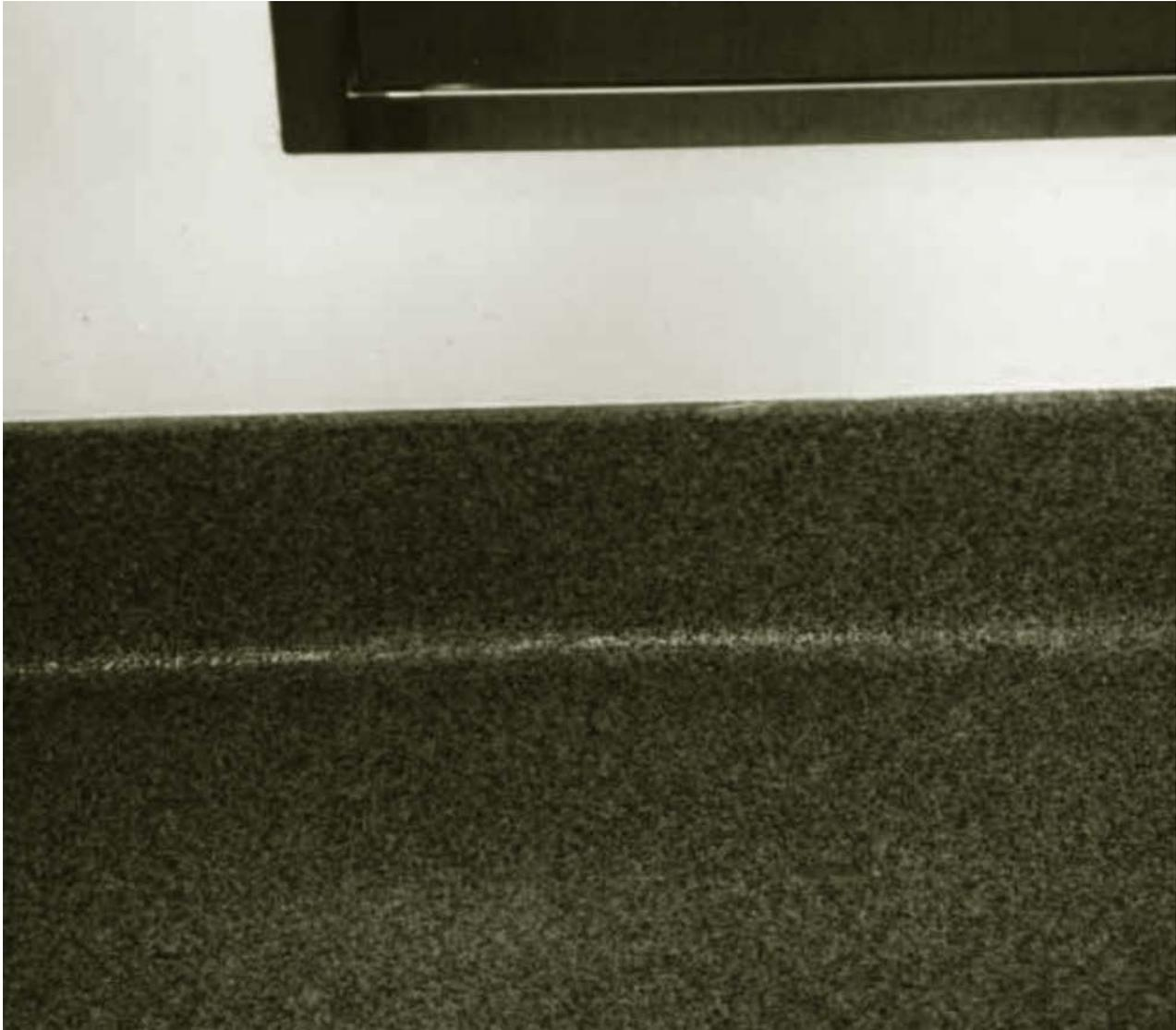
**Figure 7 depicts an example of an OR floor that extends several inches up the wall. This floor is easy to clean because dirt cannot collect at the junction of the floor and the wall.**
