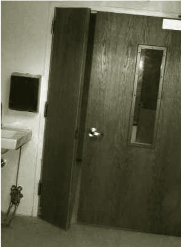
**Figure 2 depicts a two-part OR door. The main part is used for regular stretchers, while the additional section can be opened to accommodate special OR tables or extra-wide beds. Note that the wooden doors have no protection from damage by stretchers and movable equipment.**
