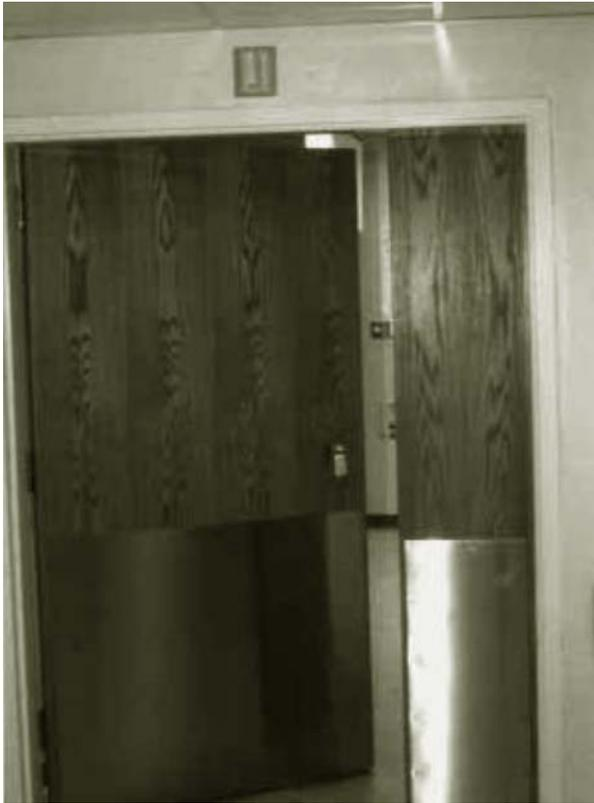
**Figure 3 depicts a two-part OR door with the addition of stainless steel overlays to protect the doors.**
