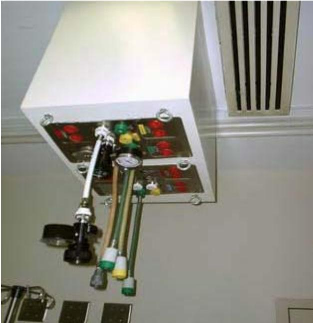
Hose connections from the wall have similar characteristics but frequently result in hoses that are lying on the floor. If wall-mounted outlets are used, then the hoses should be suspended in some manner that keeps them off the floor (or at least 3 feet away from foot and equipment travel paths).
