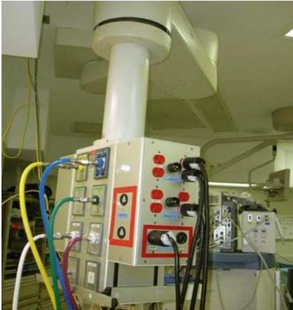
The exact location of the gas drop is critical. It is important that the hoses are not draped over the machine, damaging expensive monitors. Instead, the hoses should hang freely behind the machine and still allow personnel to walk behind it.
