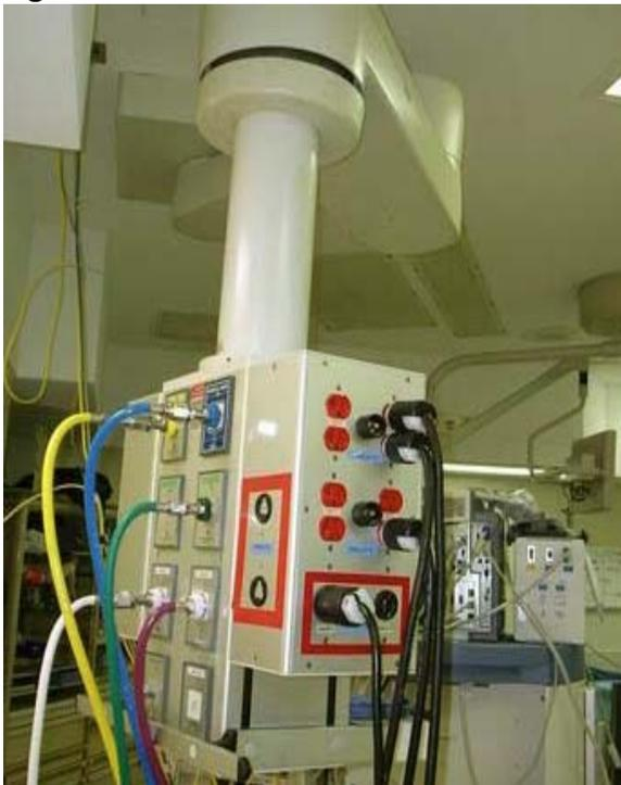
The electrical outlets can have either the standard three-prong or twist-lock type connectors. Virtually all hospital electrical equipment comes with three-prong plugs. Twist-lock plugs were an older replacement for explosion-proof connectors that were required in the days of flammable anesthetics. Twist-lock plugs provide some protection against accidental disconnection.
